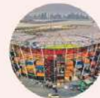
Stadium 974 The stadium of 40,000-capacity is built out of 974 shipping containers on Doha's waterfront.
